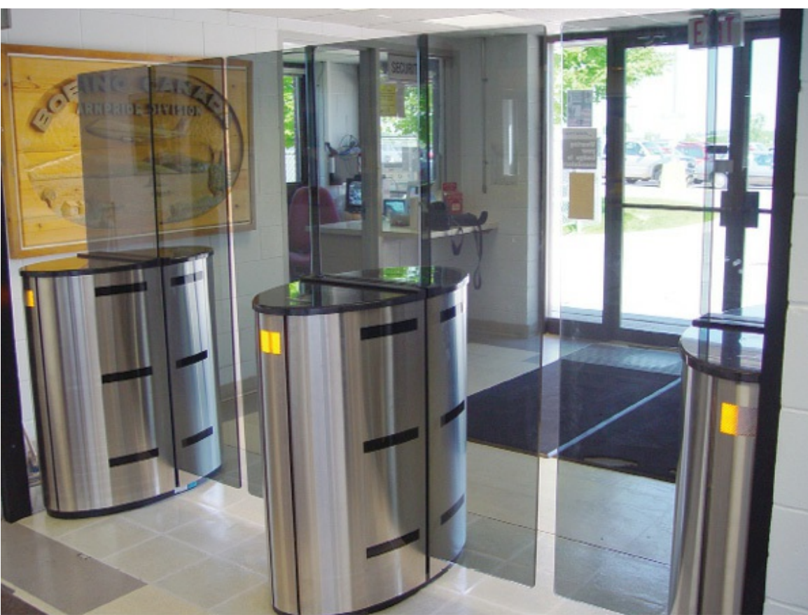
Figure 7.28 – A higher end turnstile is an optical turnstile, which is designed to provide a secure access control in the lobby of a busy building.
