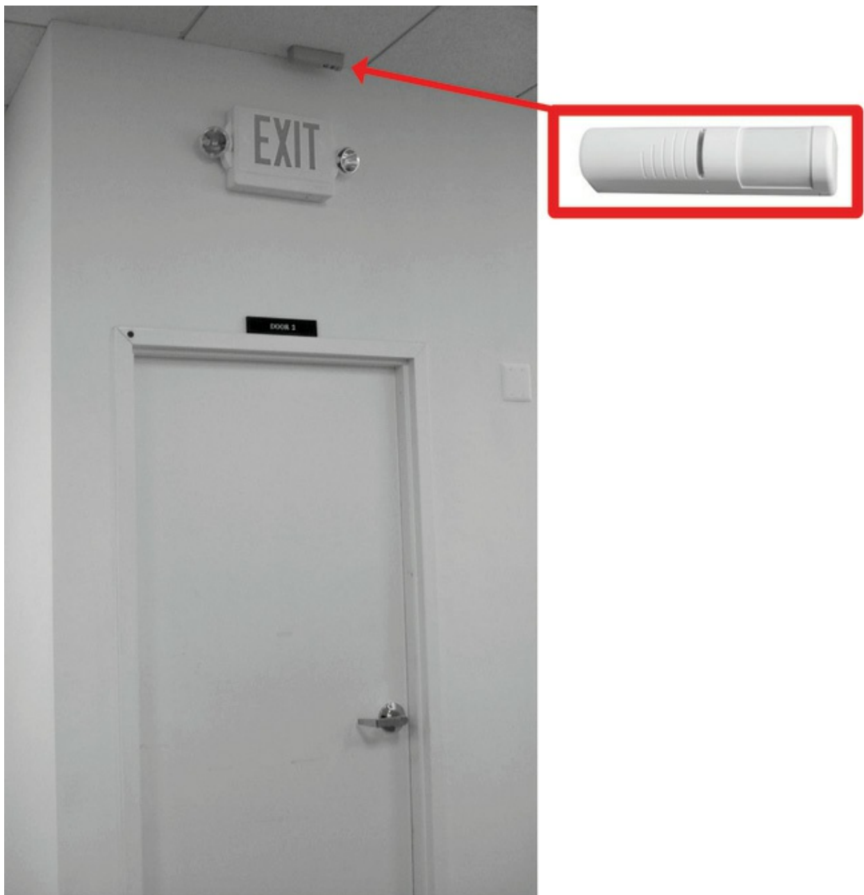
Figure 7.24 – An automatic Request to Exit (REX) device [located over the Exit sign] provides for magnetically locked doors, acting as an automatic sensor for detecting an approaching person in the exit direction and deactivates the alarm as the person exits.
