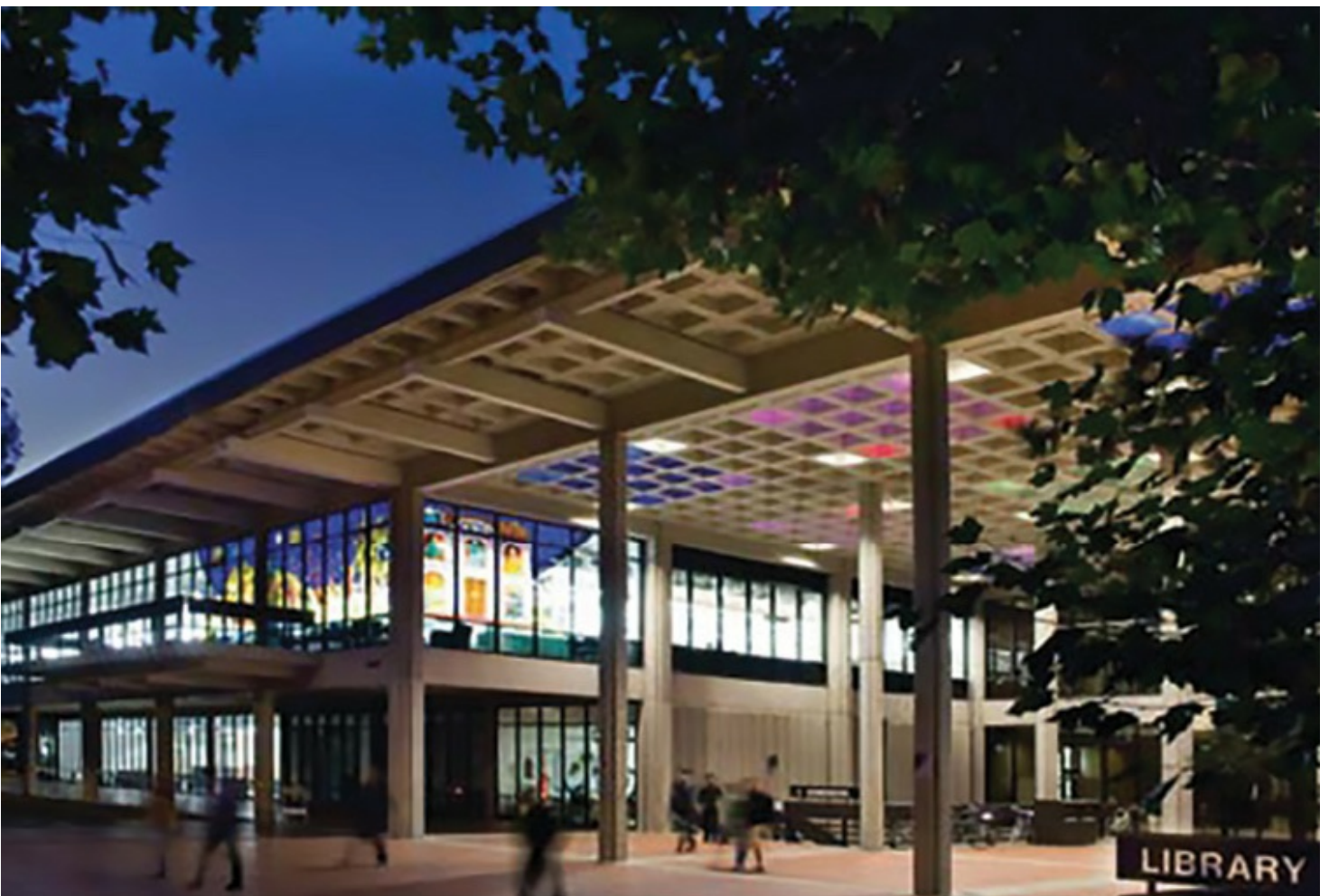
Figure 3.47 - Building designed with crime prevention in mind (Courtesy of Bosch Security Systems)
