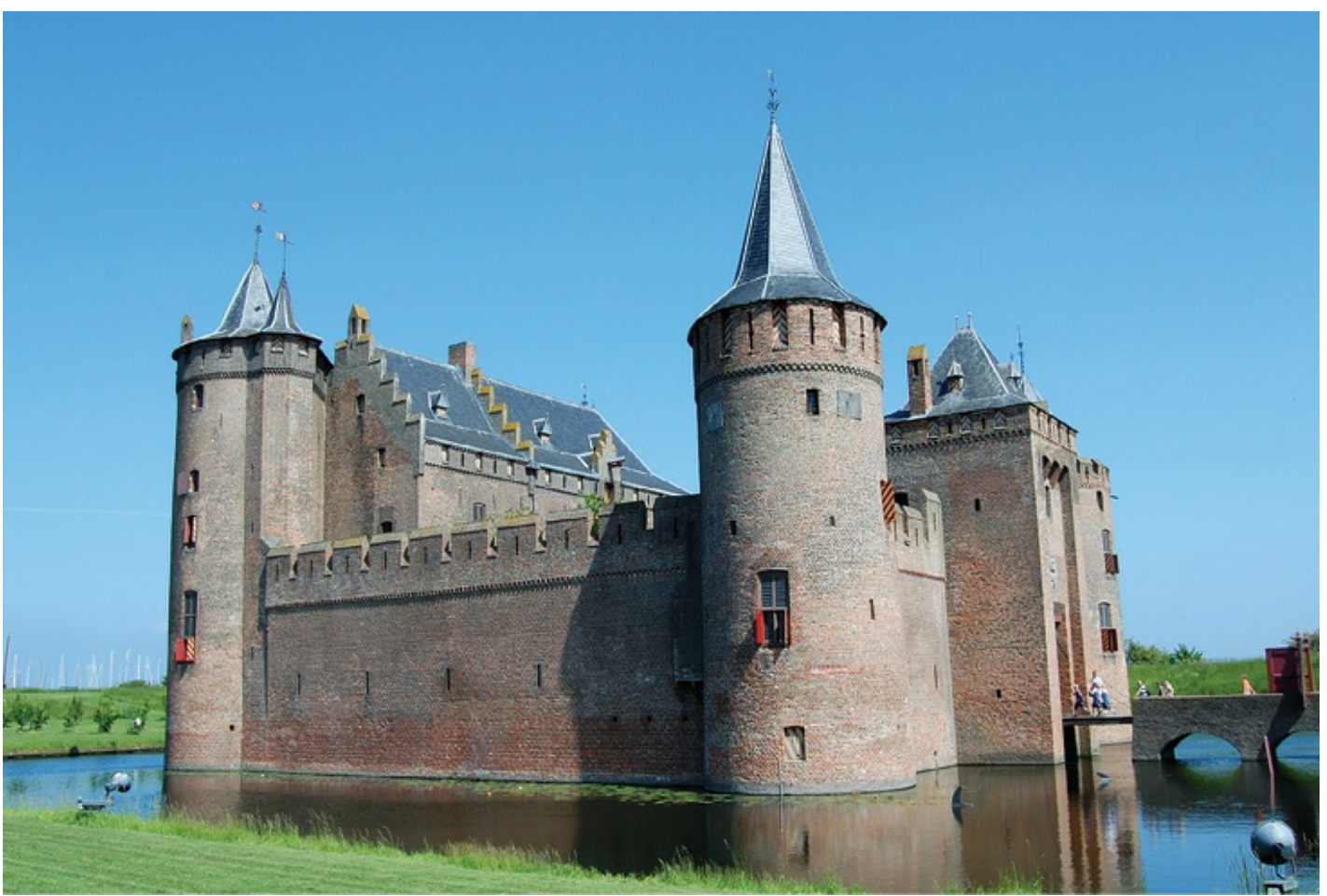
Figure 3.46 - Facility designed by a security professional (Courtesy of Bosch Security Systems)
