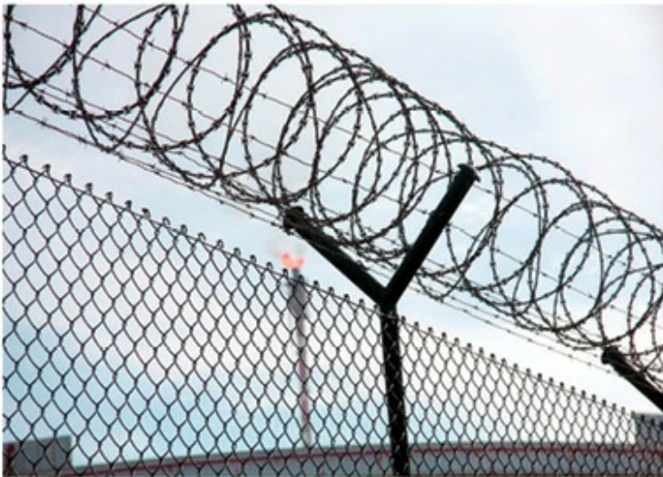
Figure 7.10 – From left to right: Ornamental fence, security fence with 3 strands of barb wire, high-security fence with 3 rolls of razor wire, and another view of rolled razor wire
